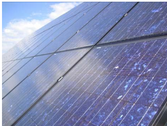
Solar Panels on the Behavioral Sciences building
